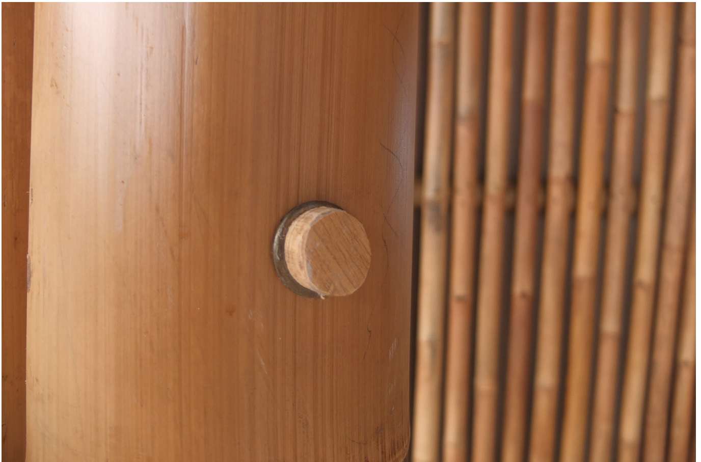
Cover of the steel bars with bamboo caps – Yoga Shala, Joali Being, Bodufushi, Maldives, 2021.
