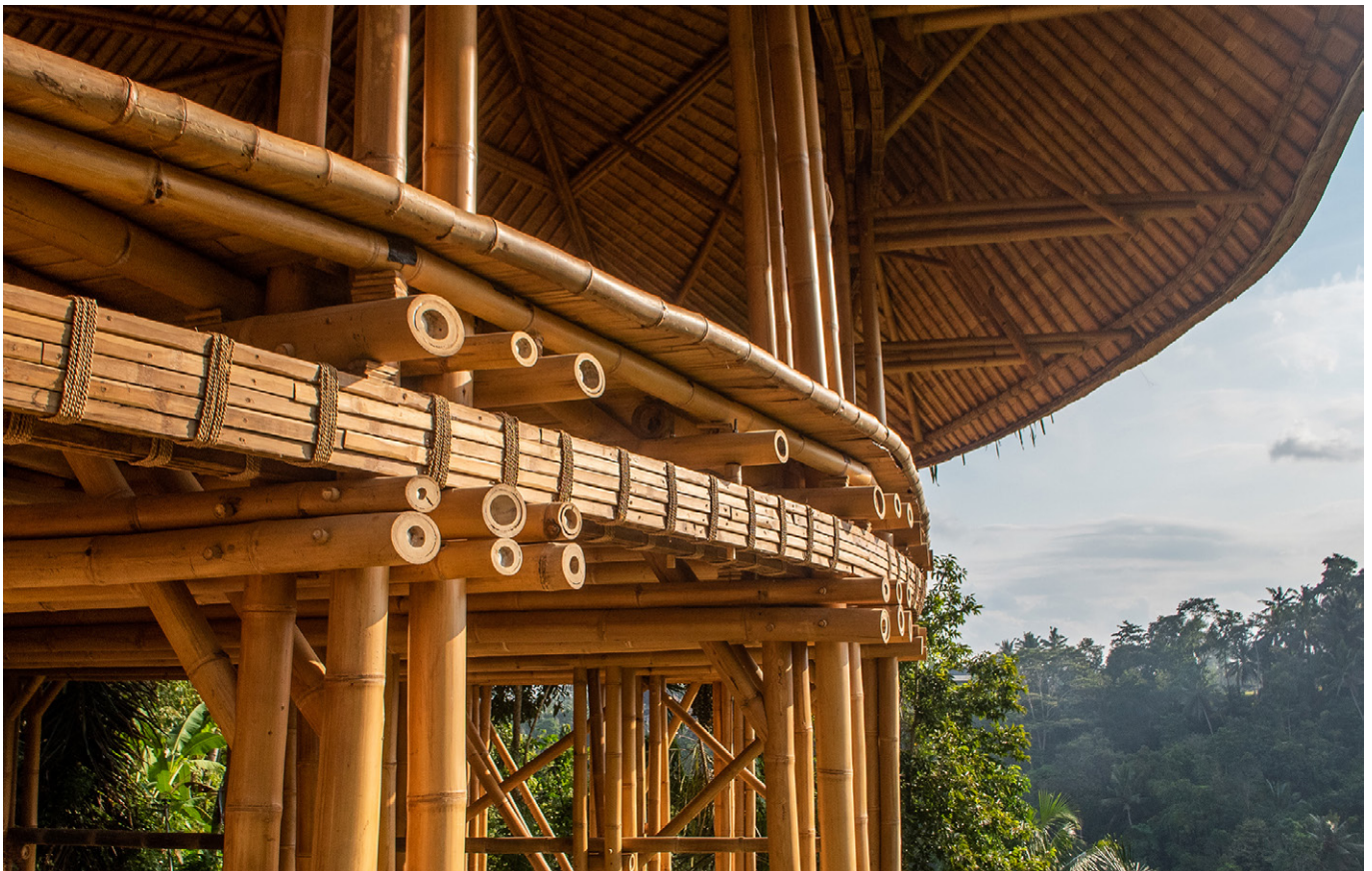
Split 5cm width without skin for bamboo split beam. During construction - Tea House, Ubud, Bali. 2020.
