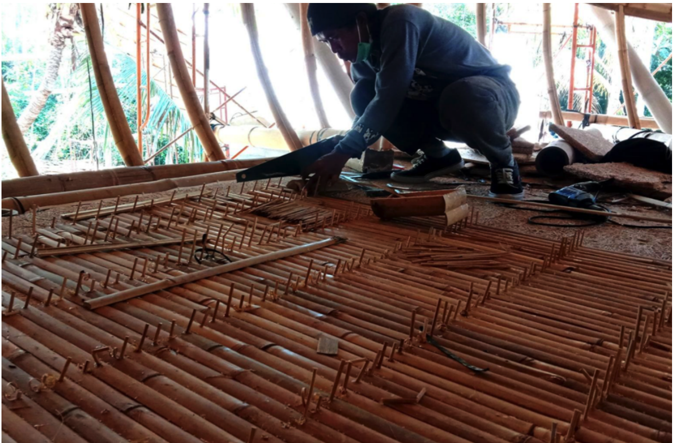
Bamboo pins Ø 4mm installation for bamboo flooring, Ulaman Eco Retreat, Kaba Kaba, Bali.
