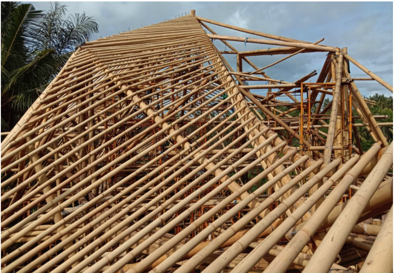
Bamboo tali poles for rafters during installation onsite. Tea House – Ubud, Bali. 2020.
