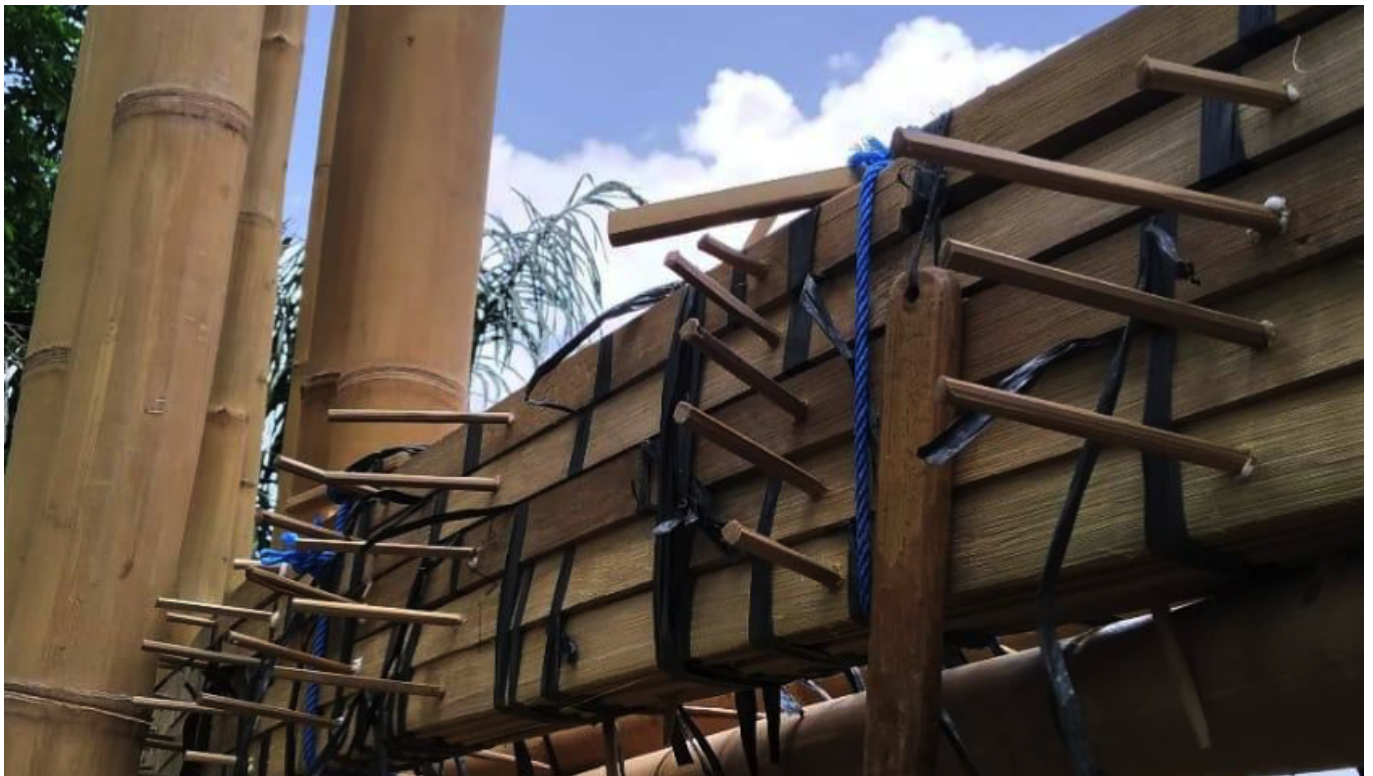
Bamboo pins Ø 8mm during installation onsite for split beam. Tea House – Ubud, Bali. 2020.
