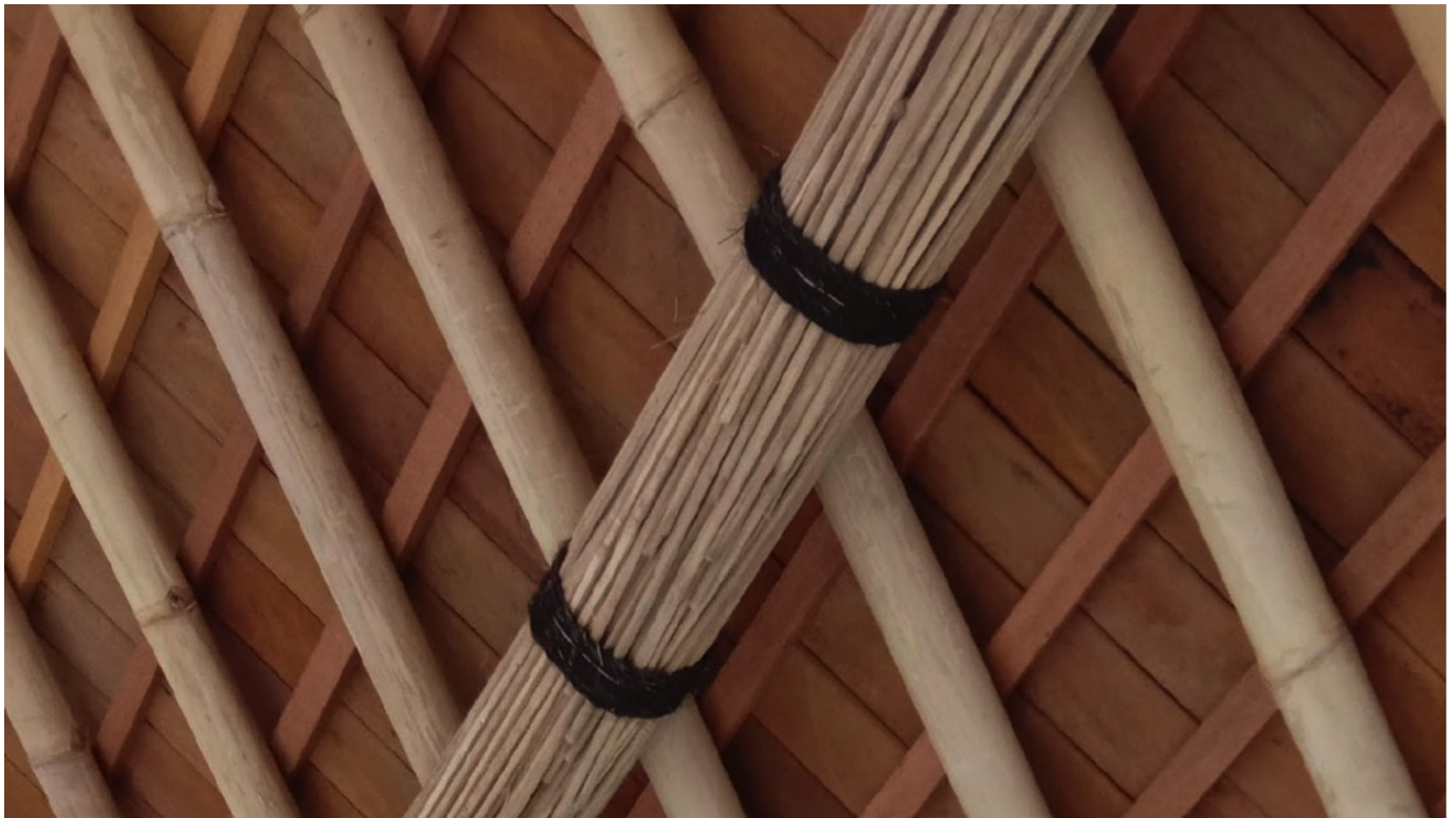
Bamboo lidi beam supporting the rafters and the roof. RASLI villa, Ubud, 2020.
