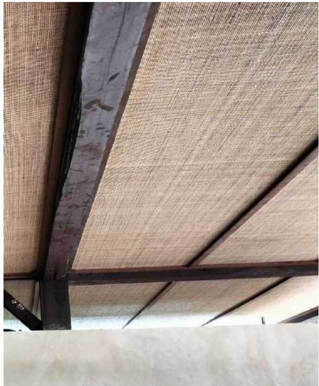
Begawan - Payangan, Bali, Indonesia 2023
